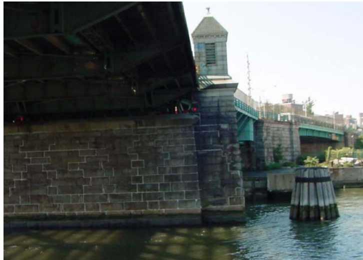
Figure 3 Masonry Blocks and Mortar Joint Pattern at West Rest Pier
